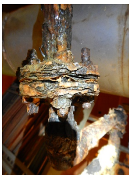
Extreme corrosion prior to Technowrap solution
