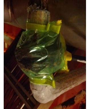
Live leak seal steps
