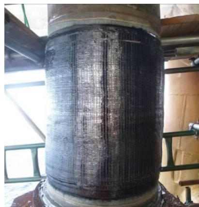
Technowrap™ repair partially completed
