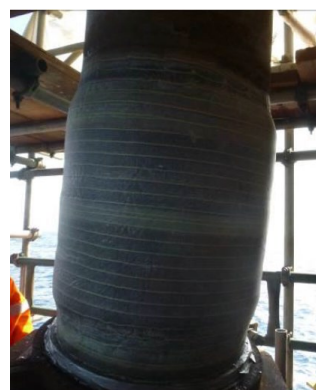
Completed Technowrap™ repair with 2k fibre final coating
